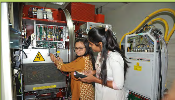
Measuring the voltage from the SMPS of a Linear Accelerator
